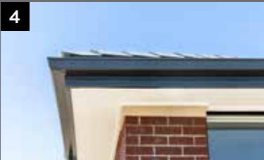
Colorbond fascia and gutter.
